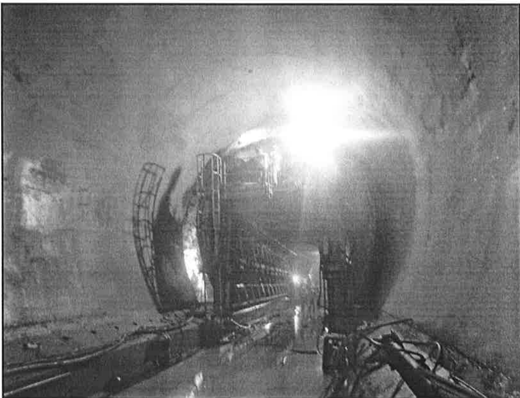
Gantry under concreting
