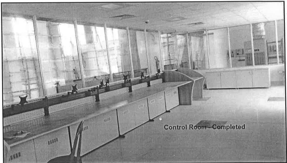
Power House Control Room
