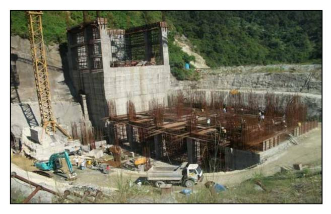
Power house - Formwork & reinforcement work in advanced stage for concreting slab
