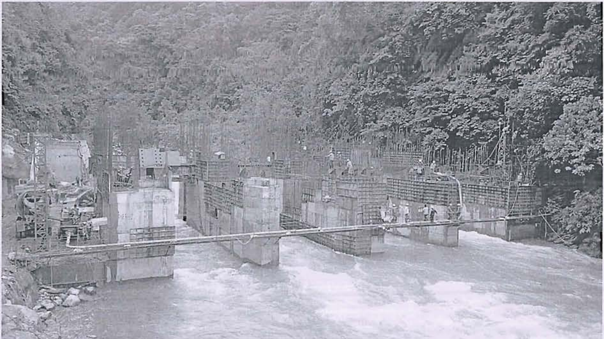
View of Barrage – Work on all piers in progress
