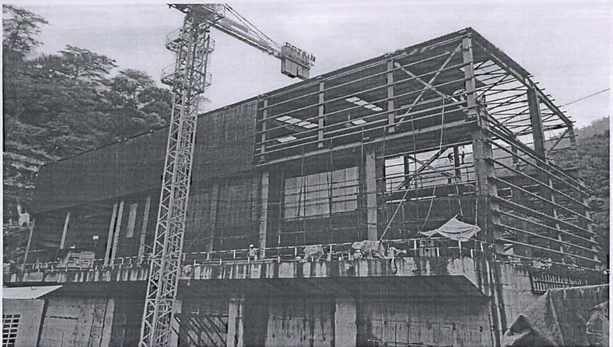
View of Power House-Purlins fixing under progress
