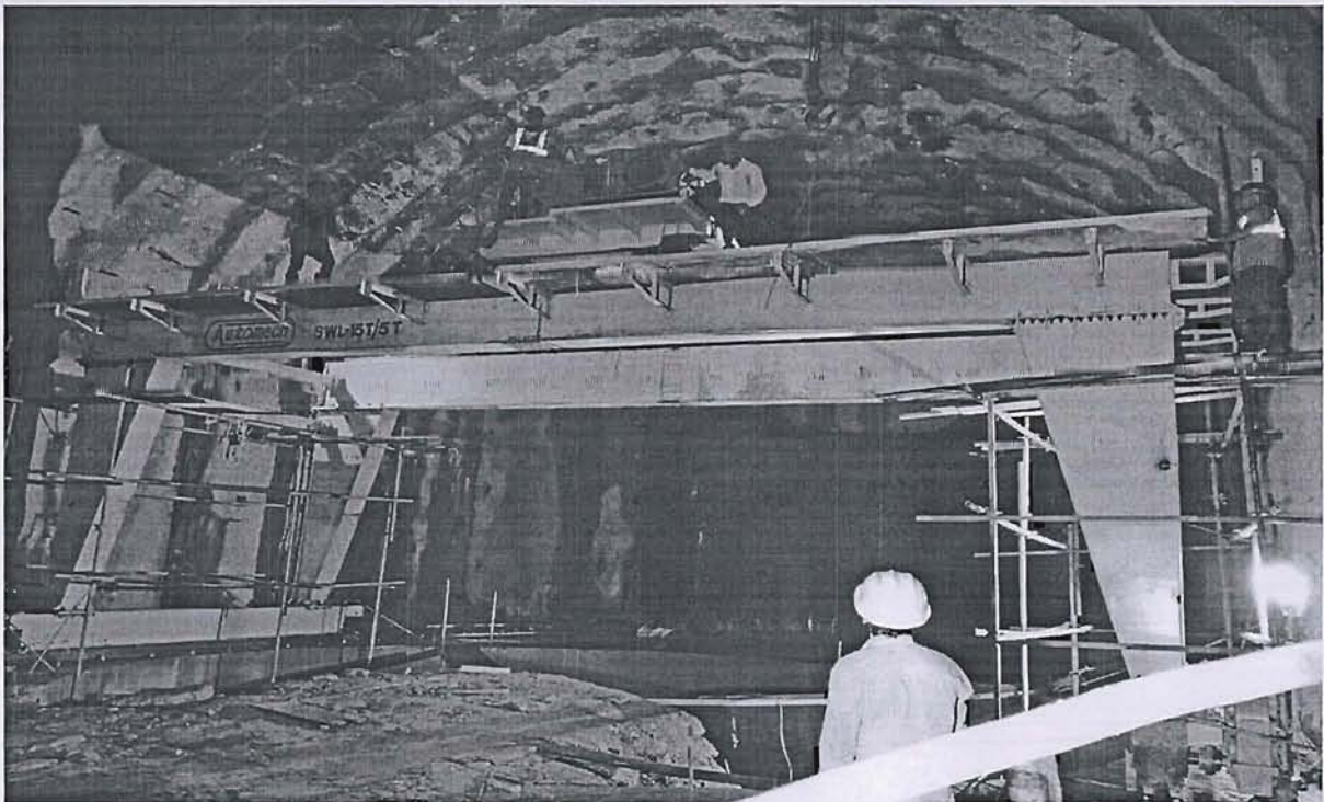
Surge Shaft Dome-Gantry Erection work under progress
