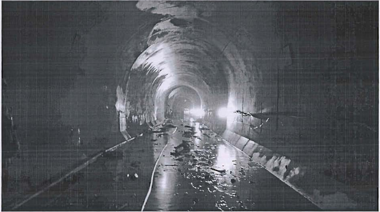
View of HRT-After Pouring Concrete
