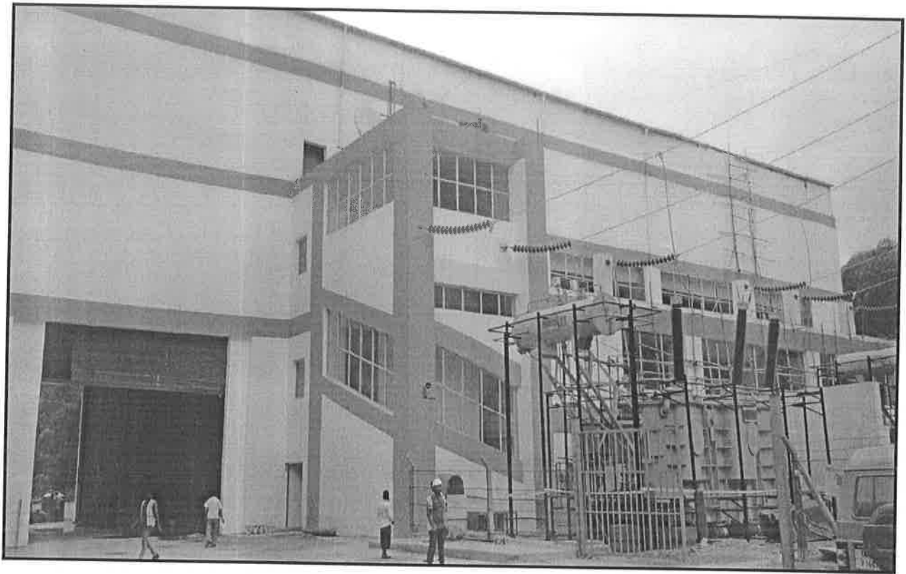
Power House U/S View
