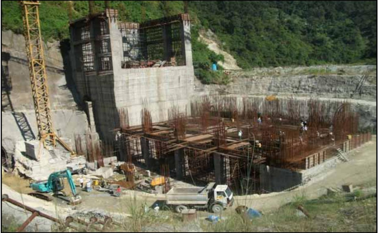
**Power house - Formwork & reinforcement work in advanced stage for concreting slab**
